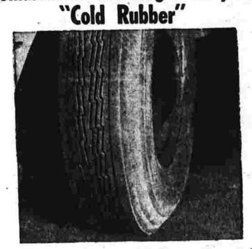
7.60-15 Tire With "Cold Rubber" Tread 521/2% of Original Tread After 21,852 Miles! sure tire with tread of 100% Cold
